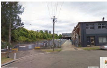
View of site looking along western boundary
